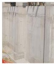
The substrate should be thoroughly cleaned from any possible formwork oil residues, loose particles, dust etc.
