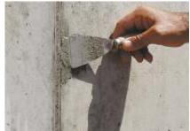
Externally, any cavities in the concrete should be cleaned from loose particles, aggregates etc. Form wires and distance pieces should be cut at a 3 cm depth. Any working joints should be widened in a V-shape along their length, at a depth of 3 cm. The surface of the above areas should be thoroughly dampened and filled with polymer modified cement mortars **DUROCRET, DUROCRET-PLUS** or **DUROCRET-FAST**.
