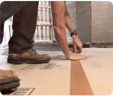
When using on a curing concrete slab, use Ram Board with our exclusive Vapor-Cure® Tape for the seams. Our Vapor-Cure® system will not only protect the slab, but promote even curing as well.
